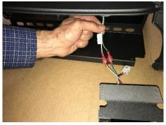
3 Remove clear plastic film from the Velcro strips on the bottom of the heatshield for the receiver. Turn the assembly over so the strips are facing downward. Gently push the wires back into the appliance as you move the receiver assembly into place. Adhere the assembly to the floor of the controls area of the stove. Make sure the placement does not obstruct the movement of the door.
