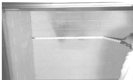
Figure 1 Measure Firebox
